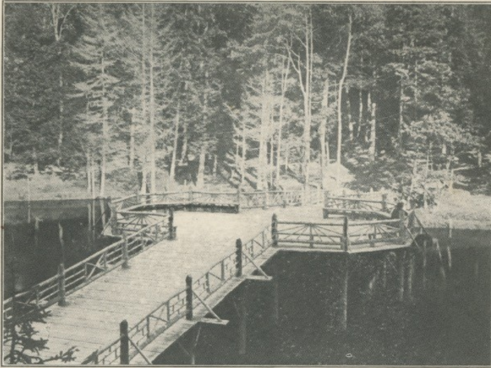
No. 53. Bridge over the Pond, Merrymeeting Park. PUB. BY F. E. MERRILL, FREEPORT
